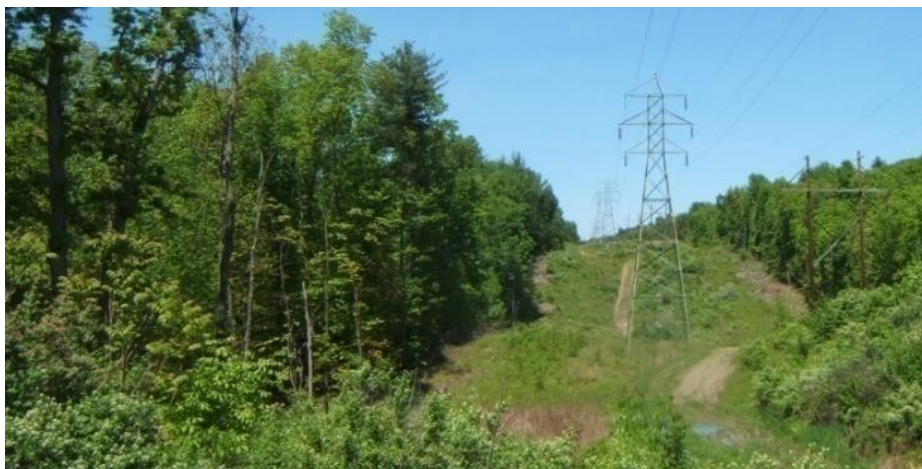
Utility right of way East of Interstate 87
