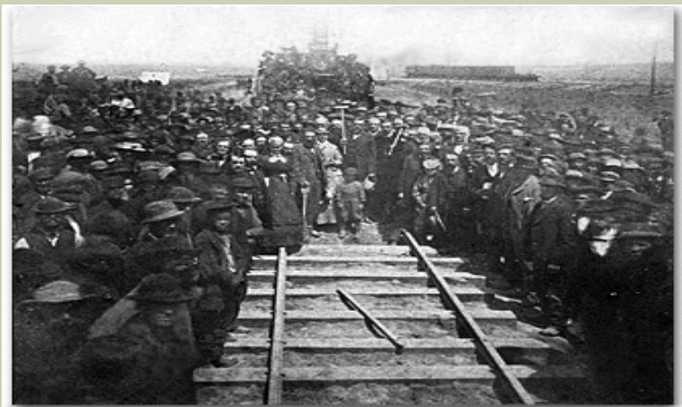
The Last Rail is Laid
